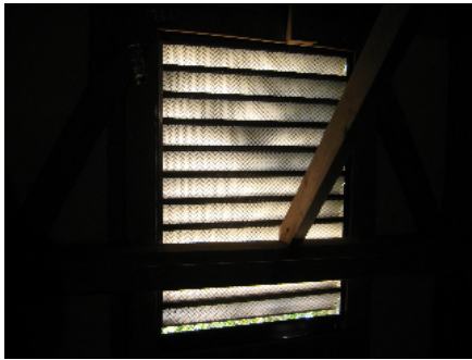
Attic Vent from inside
