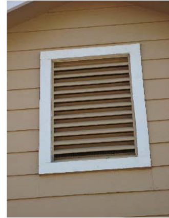
View of Attic Vent from outside
